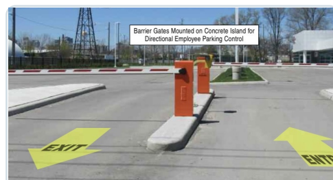
ENTRY / EXIT LANE CONFIGURATION
